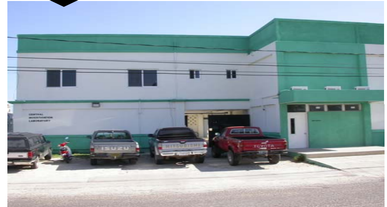
BAHA's Central Investigation Laboratory (CIL) Complex on St. Joseph Street Belize City, Belize
